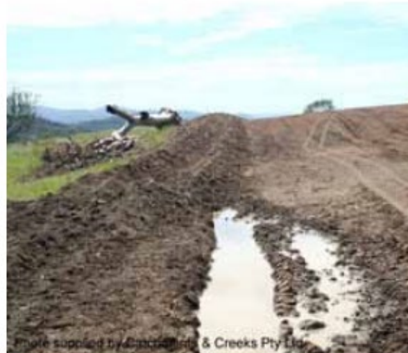
Flow diversion bank
